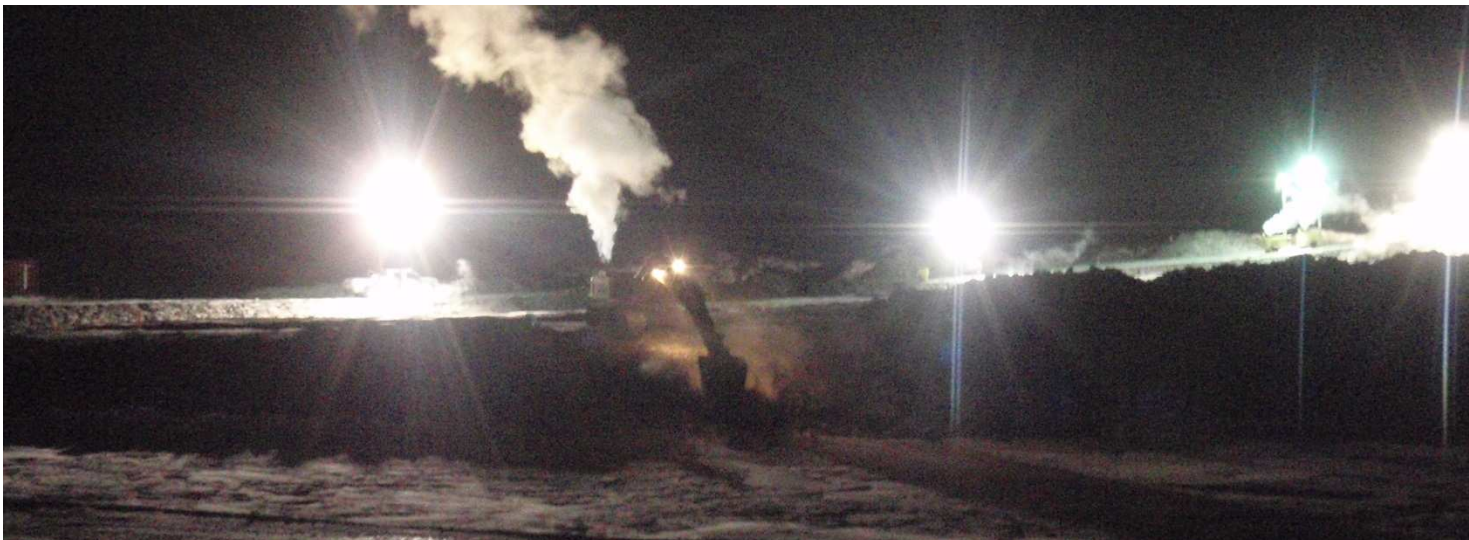
Photo 10: ~S view of excavator spreading ROQ on downstream slope to 4H:1V.
