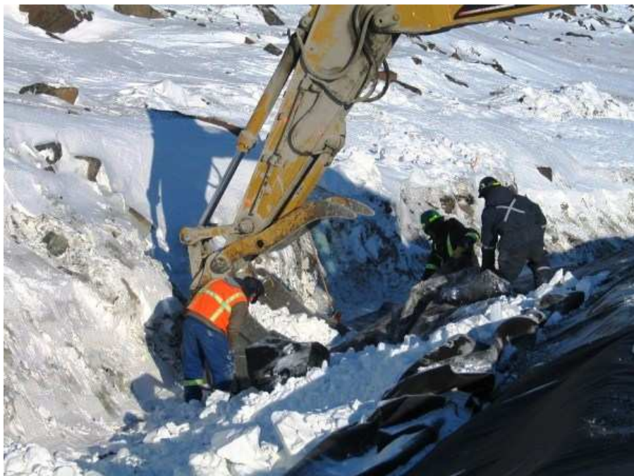
Photo 8: Liners that were cut during snow clearing.
