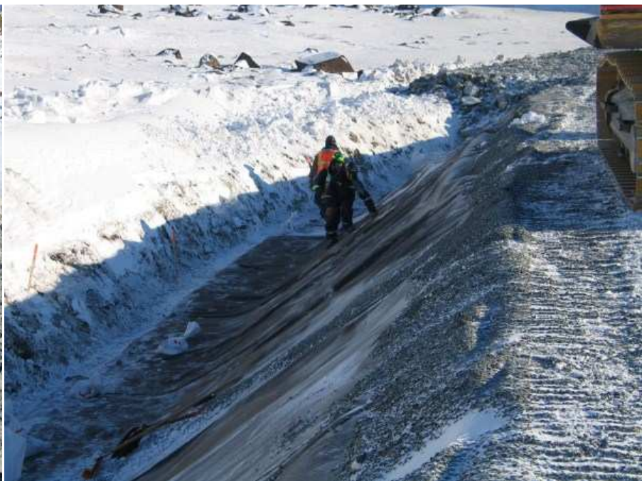
Photo 7: Labourers cleaning key trench prior to placing bentonite.
