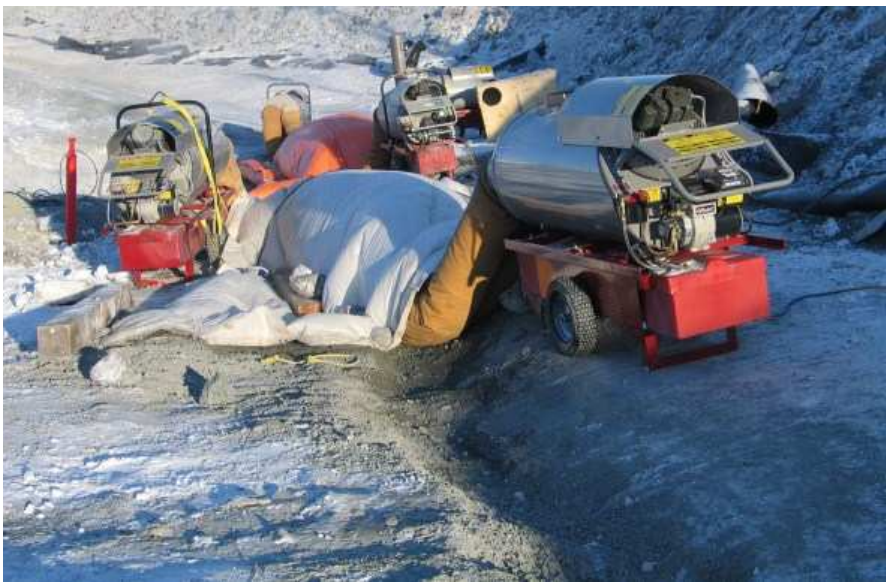
Photo 5: Frost fighters at south east corner of key
