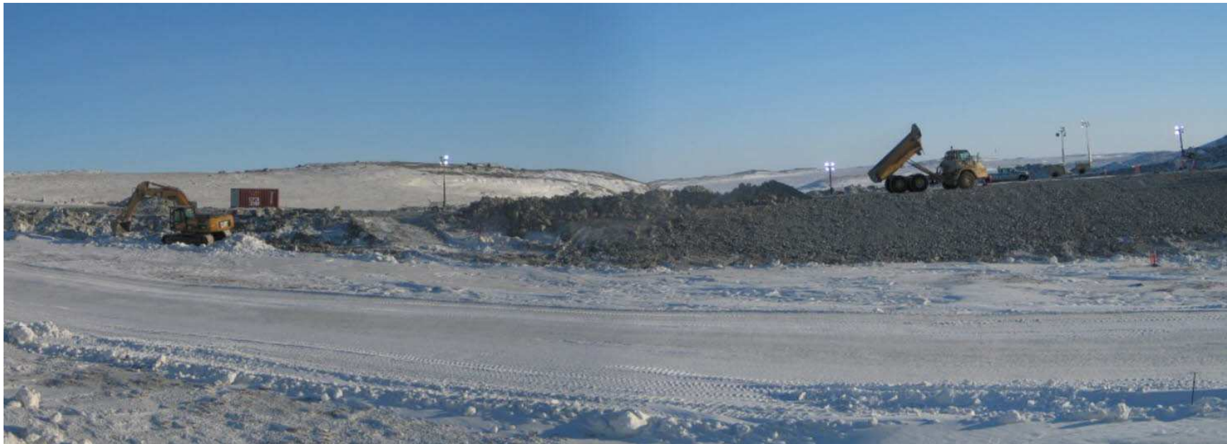
Photo 2: Panorama of downstream slope. Sloped and shaped section is between Sta 40 and Sta 1+30 Excavator is working towards north thermosyphons.
